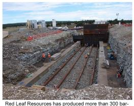
rels from its pilot capsule that tested ore from its oil shale mine in the Uinta Basin. This 2009 photo shows the capsule under construction on state land where Red Leaf heated kerogen-bearing ore to 725 degrees for seven months. Hot gas runs through the pipes and heats up the enclosed capsule like a convection oven.
